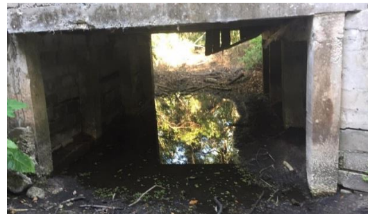
Photograph 2-4 Spring Branch South of Knollwood Drive
