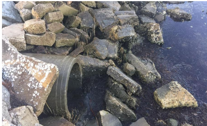
Photograph 10-2 Typical Existing Outfall Pipe to Tidal Waters
