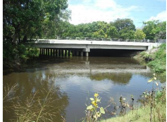
Photograph 2-2 Curlew Creek at County Road 1
