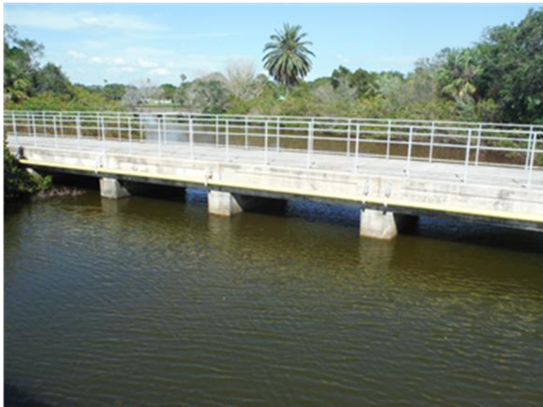
Photograph 1-2 Pinellas Trail Over Curlew Creek
